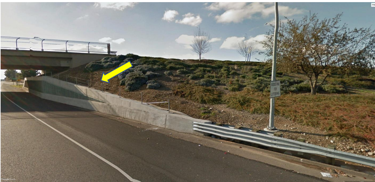
Figure 4- Retaining wall and path
